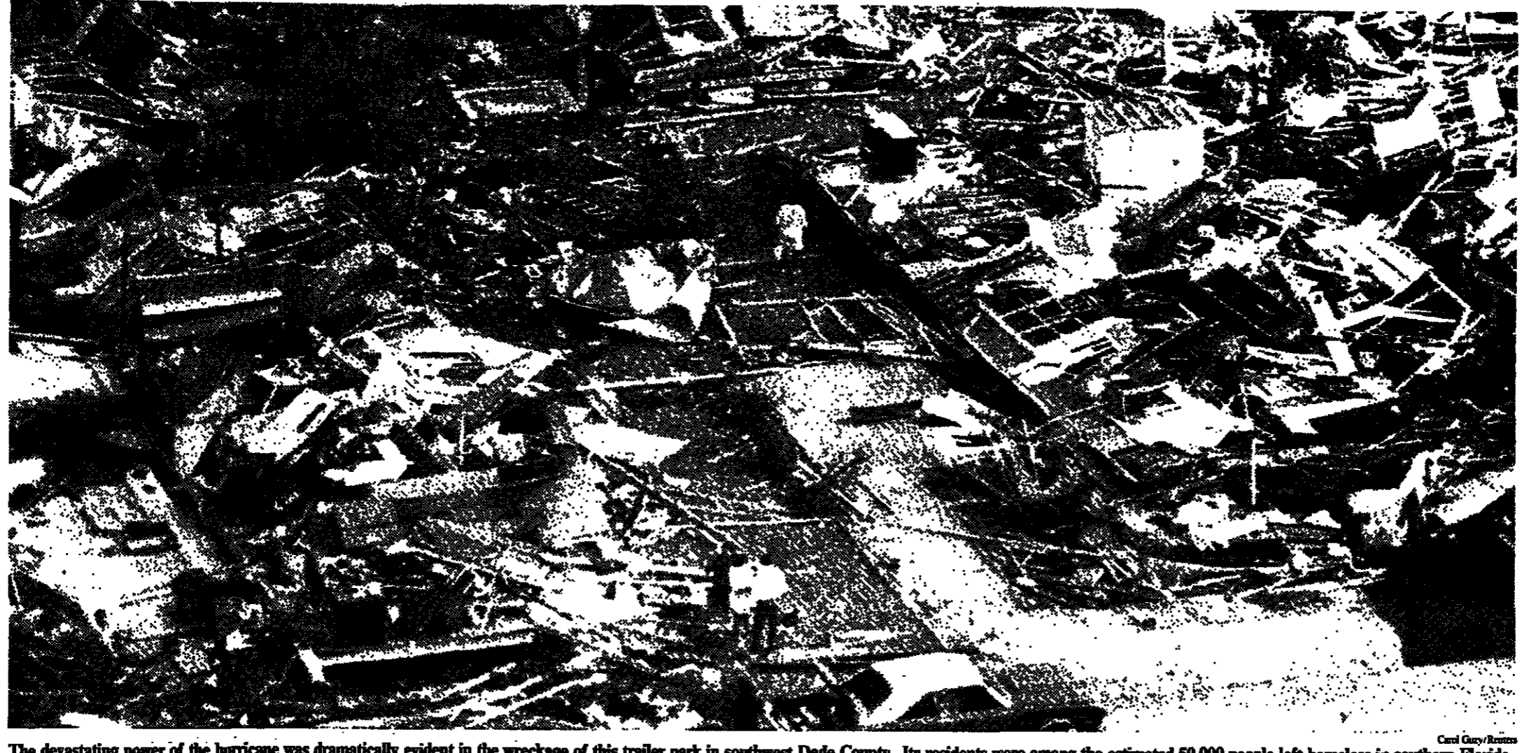
The devastating power of the hurricane was dramatically evident in the wreckage of this trailer park in southwest Dade County. Its residents were among the estimated 50,000 people left homeless in southern Florida.
